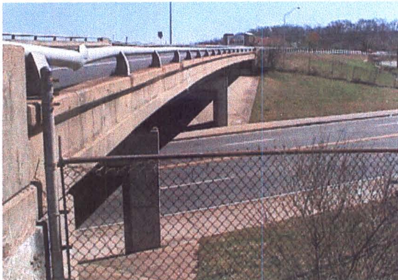
ELEVATION VIEW RT. SIDE LOOKING TOWARD ABUTMENT #2
