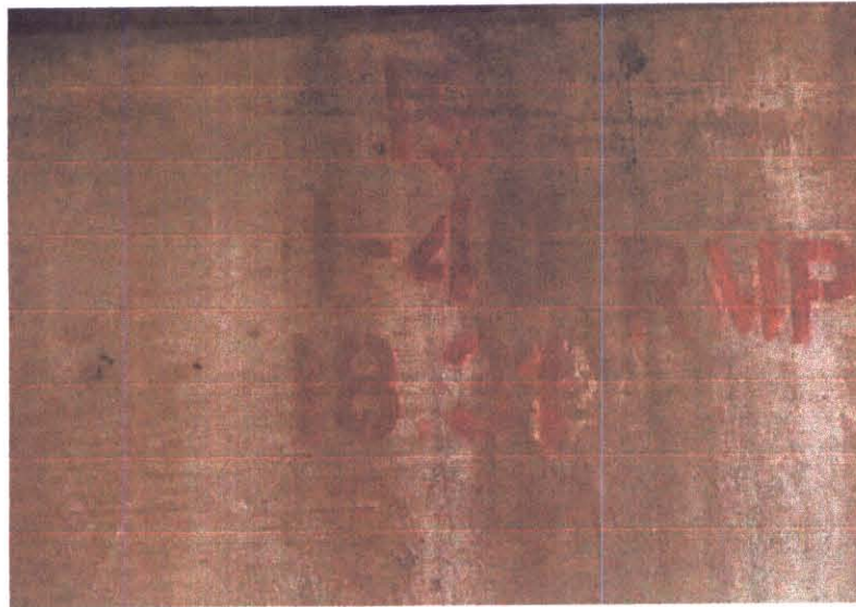
BRIDGE NO. AT ABUTMENT # 1
