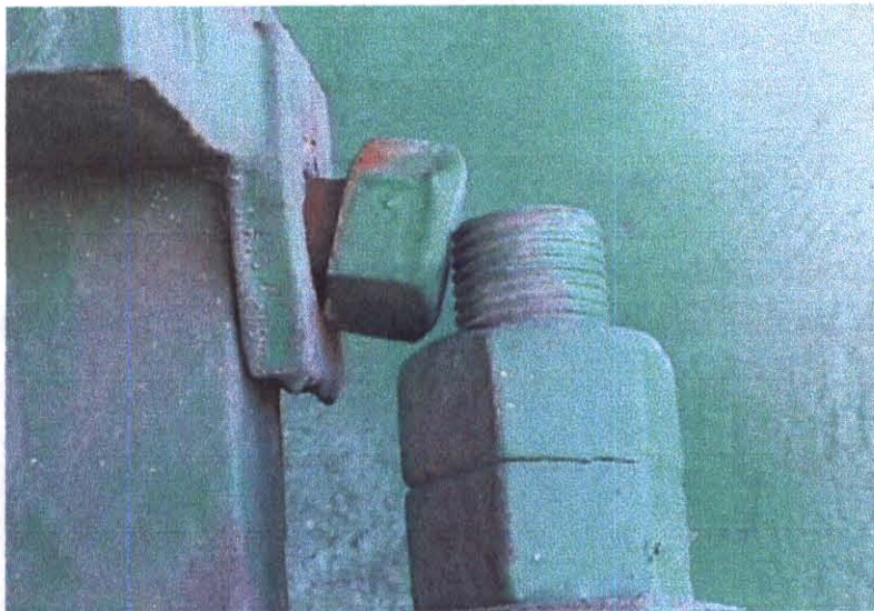
BEARING PIN BEAM "A" AT ABUTMENT #1
