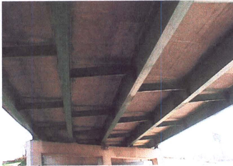
BOTTOM DECK SPAN #2 TYPICAL
